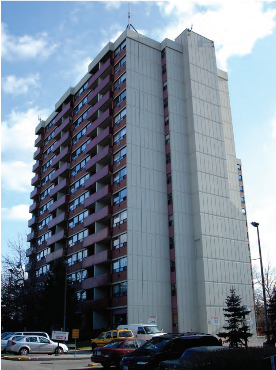
Figure 7.32. Example of a tower building where the projecting shear walls divide the balconies, serving as a separator and simplifying the balcony enclosure construction.
