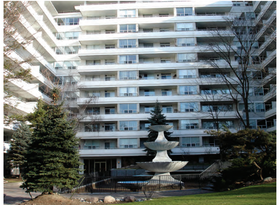
Figure 7.39. Mixed balcony arrangements are evident in this building. The balconies in the facing elevation are enclosed on one or both sides by projecting shear walls. Balconies on the side elevations are continuous and are fitted with metal partitions to subdivide the balcony space and allocate it to the individual suites.
