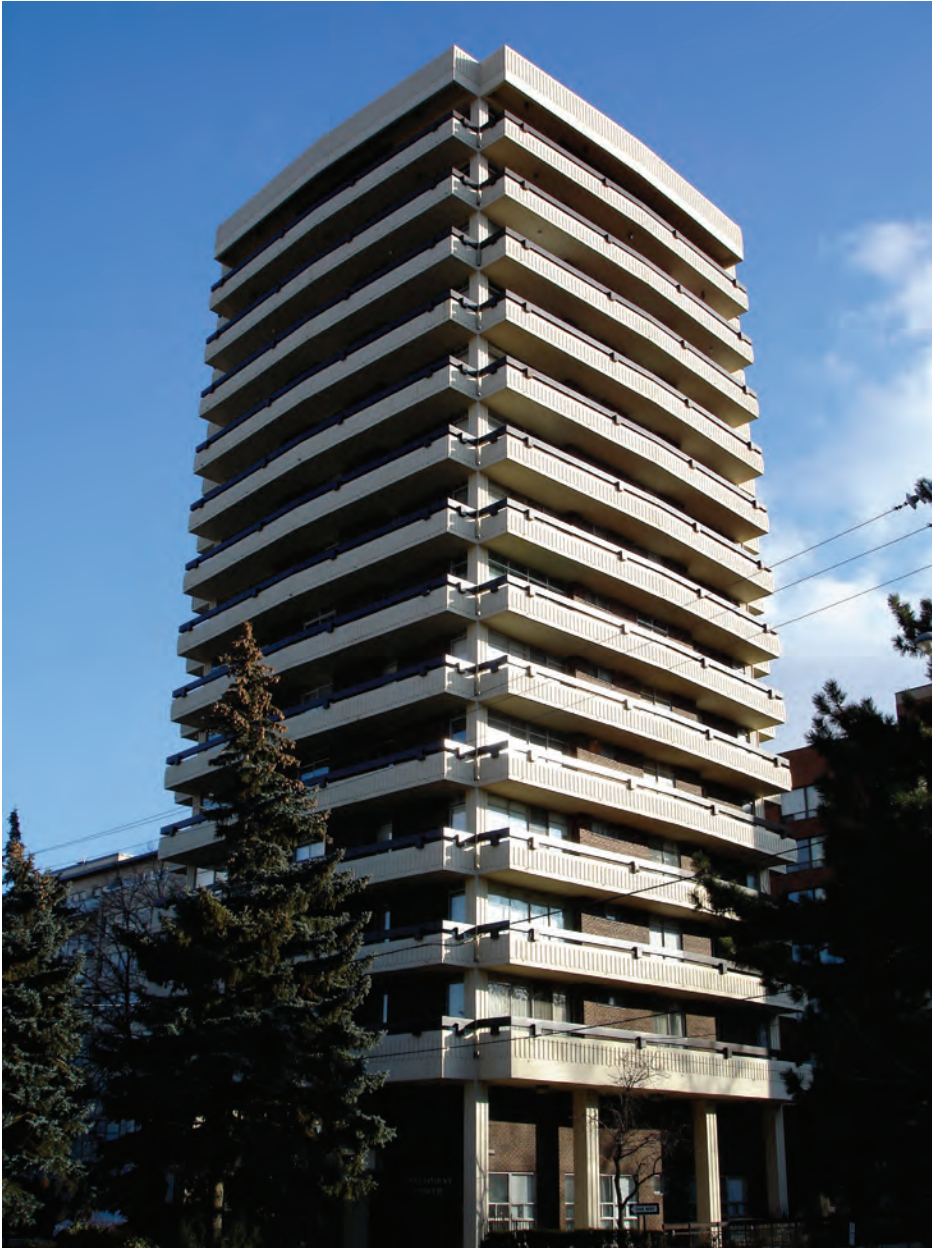
Figure 7.42. Point towers with continuous balconies and cast concrete guards, such as the one depicted above, are among the most costly to retrofit by any means.
