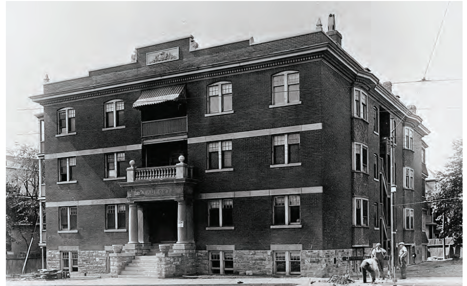
Figure 4.1. Apartment building at 359 Davenport Road, Toronto in 1931. Three and four storey walk-up apartment buildings like this one, so named because they did not provide elevators, dominated rental income housing projects. These buildings employed solid masonry walls with hybrid wood and steel interior structures. Notches were commonly set into the sides of these buildings to deliver light and air to interior rooms. [Source: City of Toronto Archives.]
