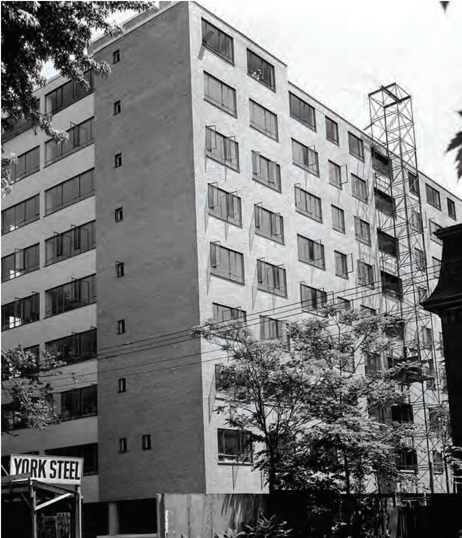
Figure 4.4. This early 1960s apartment building employs a hybrid structural system comprised of steel and reinforced concrete. There is no underground parking and minimal site parking for this urban infill development. Note the absence of balconies and the use of single glazed, steel frame windows. The small windows serve bathrooms without means for mechanical ventilation. [Source: City of Toronto Archives.]
