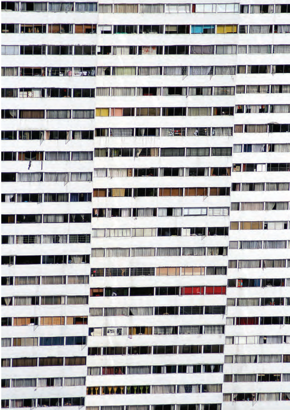
Figure 9.7. Many tower building inhabitants have no other housing alternatives. They are forced to endure retrofit work that may extend for over a year before everything is properly completed. Designers and contractors should endeavour to minimize the intrusiveness of the retrofit work being proposed. [Photo: Svenwerk.]
