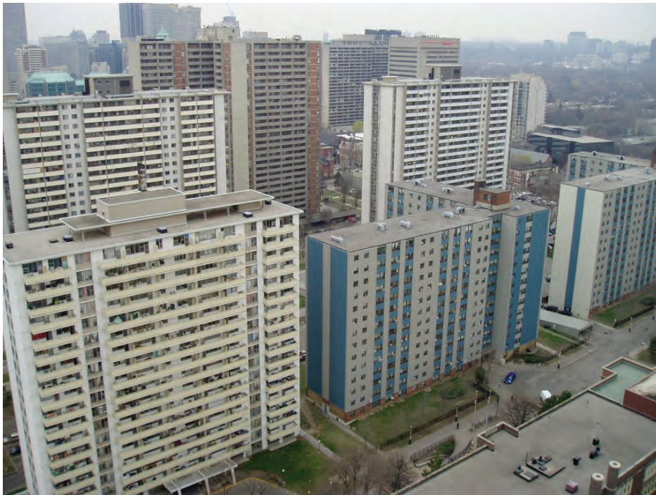
Figure 2.2. St. Jamestown in the heart of downtown Toronto is an example of an area that is intensely populated by tower buildings. Unless appropriate planning and renewal strategies are adopted, areas like this could be disrupted for more than a decade as the retrofit work proceeds from one building to another. Noise, dust and traffic congestion are among the logistical challenges associated with tower renewal in urban cores. Disparity between the inhabitants of retrofit towers and those awaiting retrofit are social challenges stemming from several decades of benign neglect. [Photo: Simon Pulsifer]
