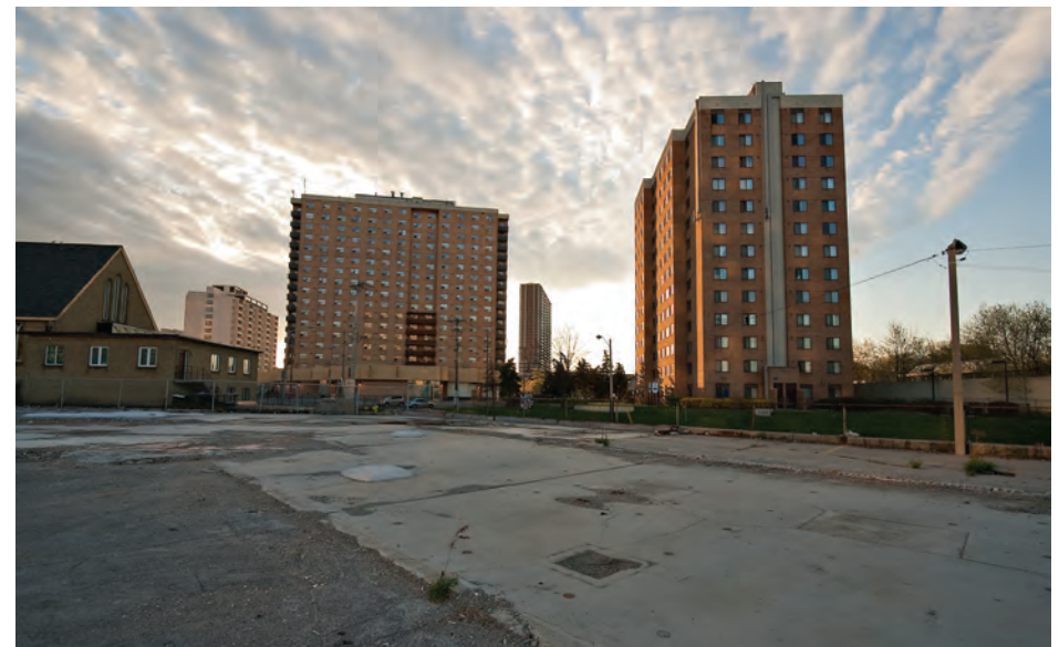
Figure 2.1. Tower renewal must also focus on the site and urban landscapes if it is to achieve its full potential. Stormwater management, green spaces and recreational amenities are essential measures that speak to environmental responsibility and inhabitant well-being. [Photo: Jesse Colin Jackson.]
