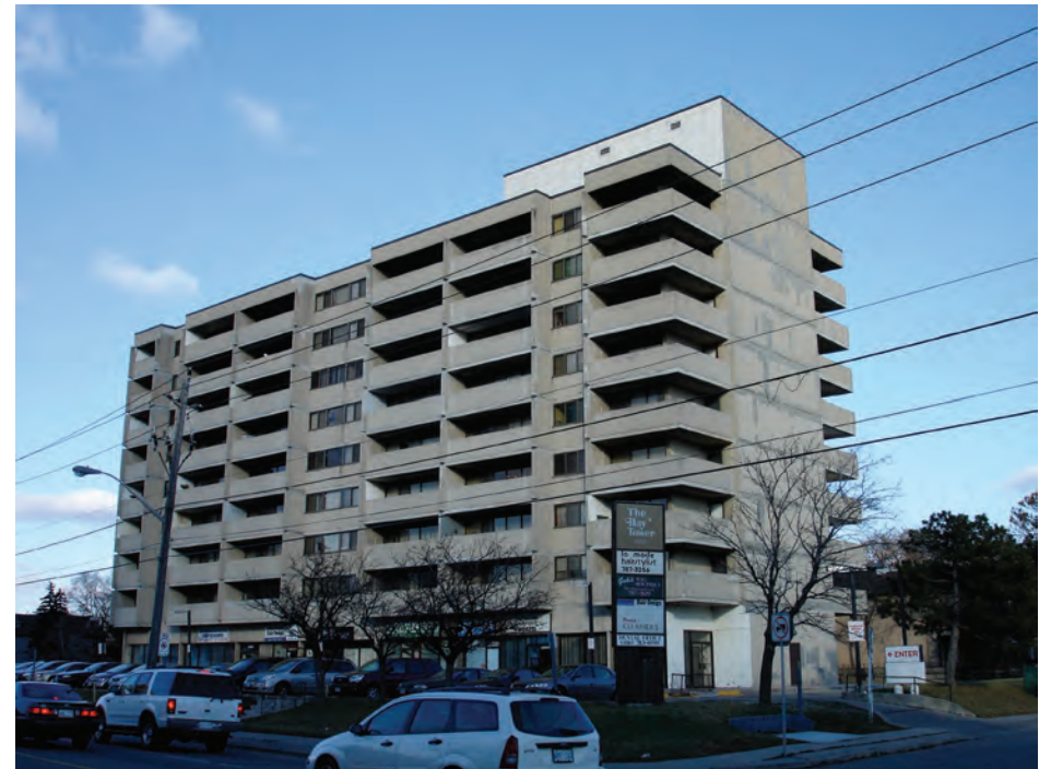
Figure 7.41. Cast concrete guards at the outside of the single balconies separated by projecting shear walls make it practically much easier to enclose these spaces and to integrate the enclosures with the overcladding.
