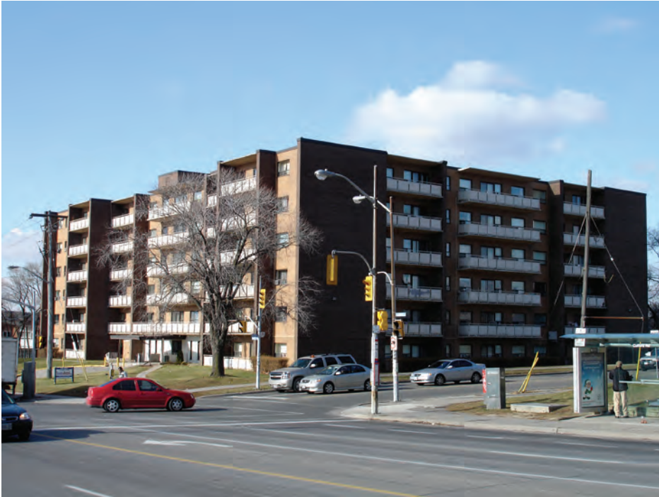
Figure 7.34. Balconies on this apartment building vary, with some enclosed on two sides by projecting shear walls, and others having all three sides open. There may be cost advantages to considering a combination of balcony enclosure and balcony overcladding strategies for this type of building.
