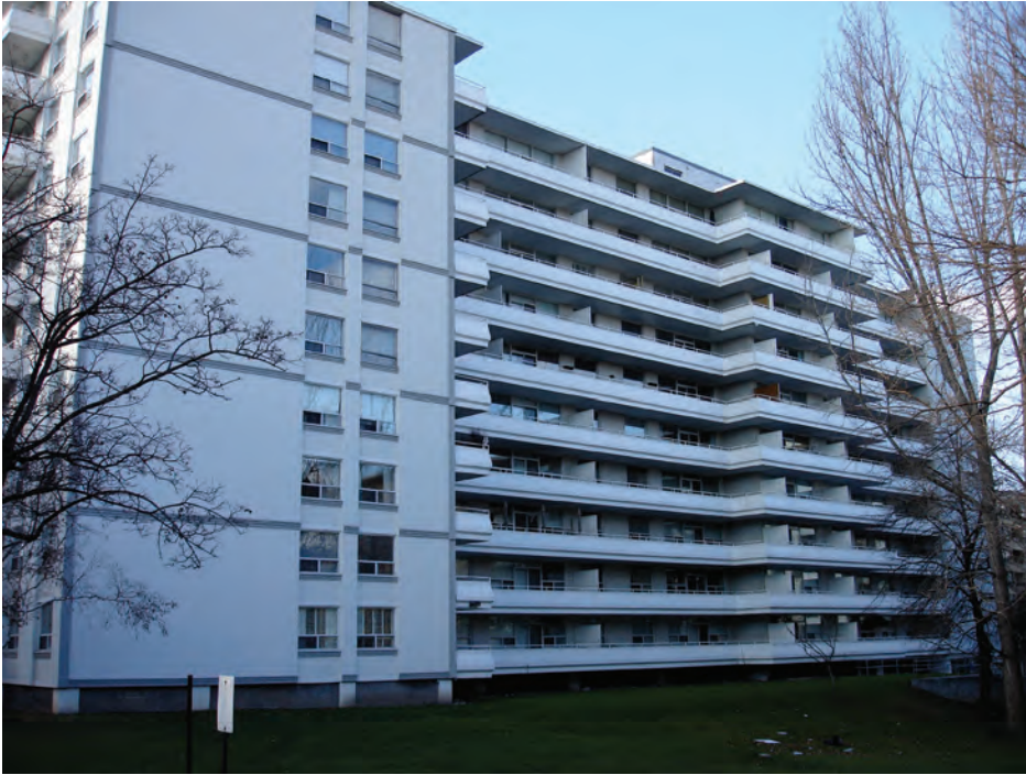
Figure 7.38. This building is an example of continuous balconies wrapping around the exterior of the building. Balcony enclosure will represent a much higher cost in this type of building than the types with individual, spaced balconies.
