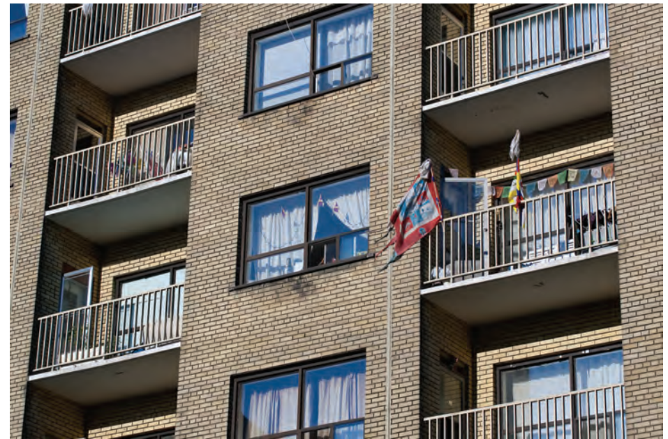
Figure 7.29. The highest potential for balcony enclosures adversely affecting daylighting and natural ventilation is associated with recessed balconies. [Photo: Jesse Colin Jackson.]
