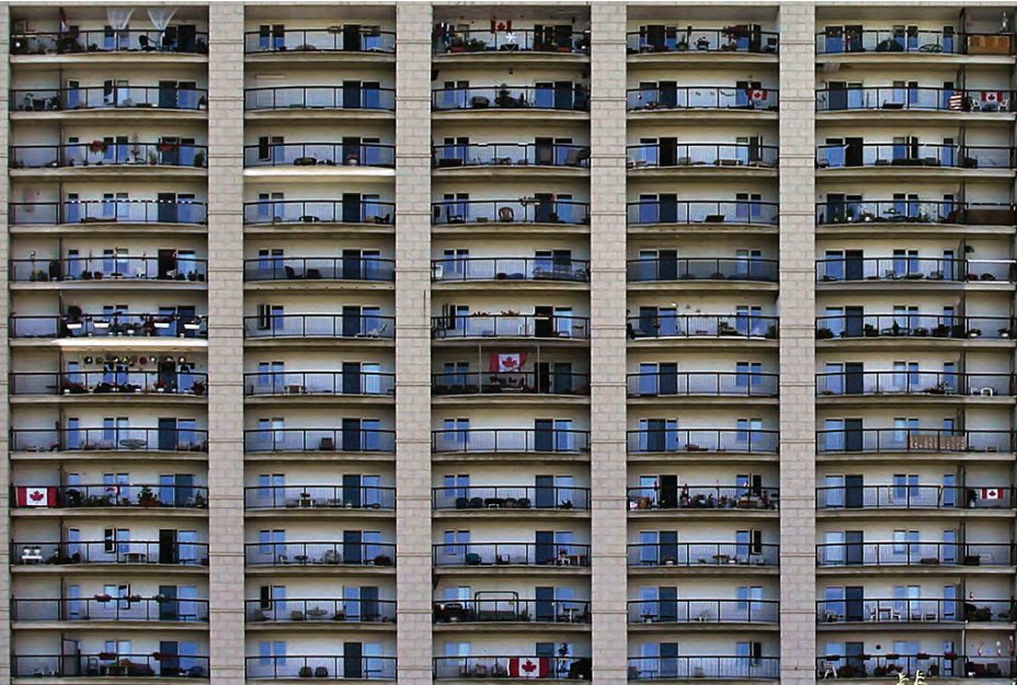
Figure 3.3. This high-rise apartment building in Winnipeg may look straightforward as an envelope retrofit, but the summer season here is much shorter here than many parts of Canada. Winter retrofit is often interrupted by inclement weather and labour productivity is lower in the cold. Weather protection and winter heating of the work enclosure all combine to add significant costs to out-of-season projects. [Photo: Daniel Hornseth.]
