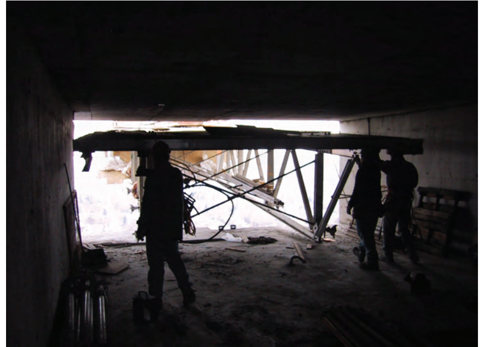
Figure 4.9. A section of flying formwork is guided out of a building bay by workers, as it is pulled from above by the climbing crane. This section will be hoisted to the floor above in preparation for the construction of the next storey of the tower building.
