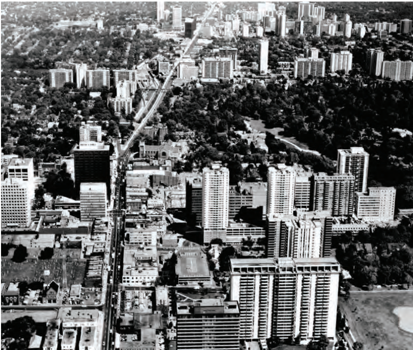
Figure 4.8. The two photos above illustrate the densification of residential neighbourhoods, spurred on by construction of the Yonge subway line in Toronto, and made possible through flying form technology. [Source: City of Toronto Archives.]
