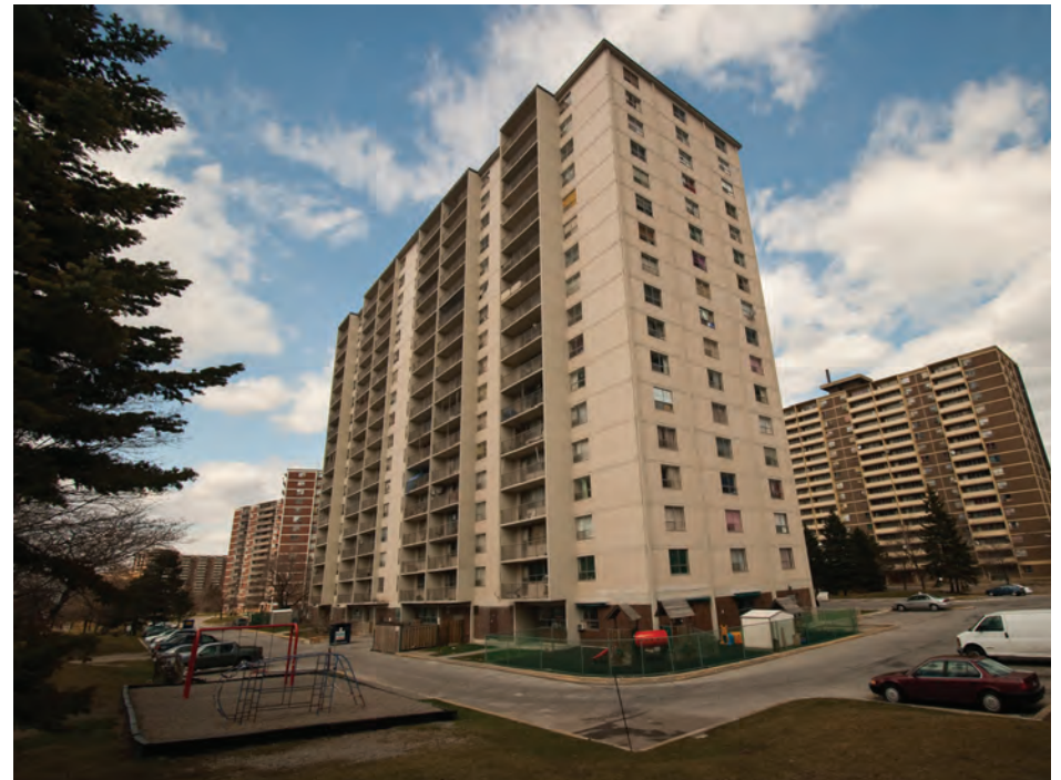
Figure 6.28. This tower building contains a daycare centre on the ground level, and represents a situation where re-location would be recommended as the most prudent means of addressing retrofit construction impacts to the inhabitants. [Photo: Jesse Colin Jackson]
