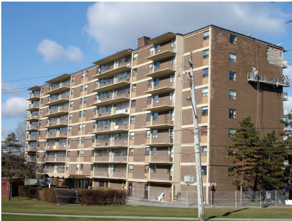
Figure 7.36. Example of a building where there is a low proportion of replacement windows in the exterior walls where overcladding will be applied. Note that the balcony guards have been removed and the doors to the balconies blocked from the outside for occupant safety. Remedial work on the existing envelope is underway before the remainder of the retrofit is performed.
