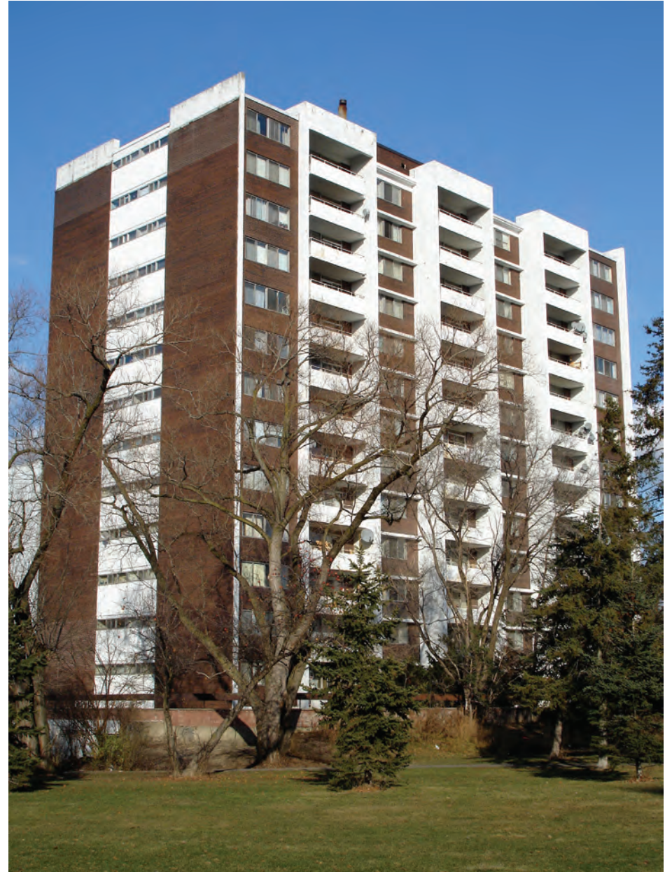
Figure 7.35. This building has balcony floor slabs spanning between projecting shear walls. Note that the balcony slabs are recessed from the outer edge of the shear walls, requiring the shear wall overcladding to be integrated with the balcony enclosure. Modest window openings on the end shear walls help make this portion of the overcladding easily executed and economical.
