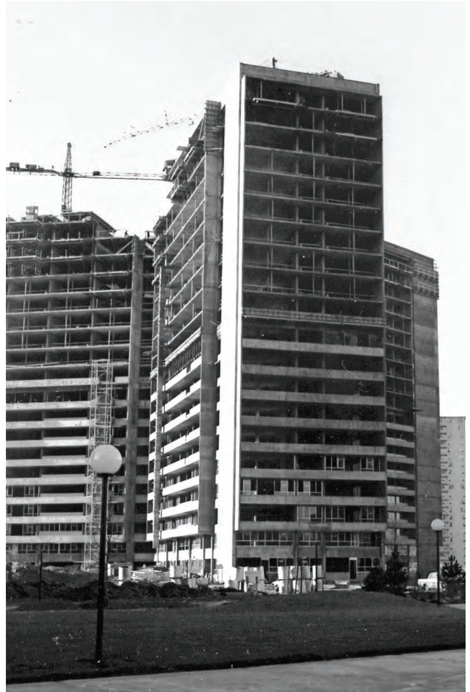
Figure 1.2. Thorncliffe Park under construction. [Photo: Archives of Canadian Architect.]
