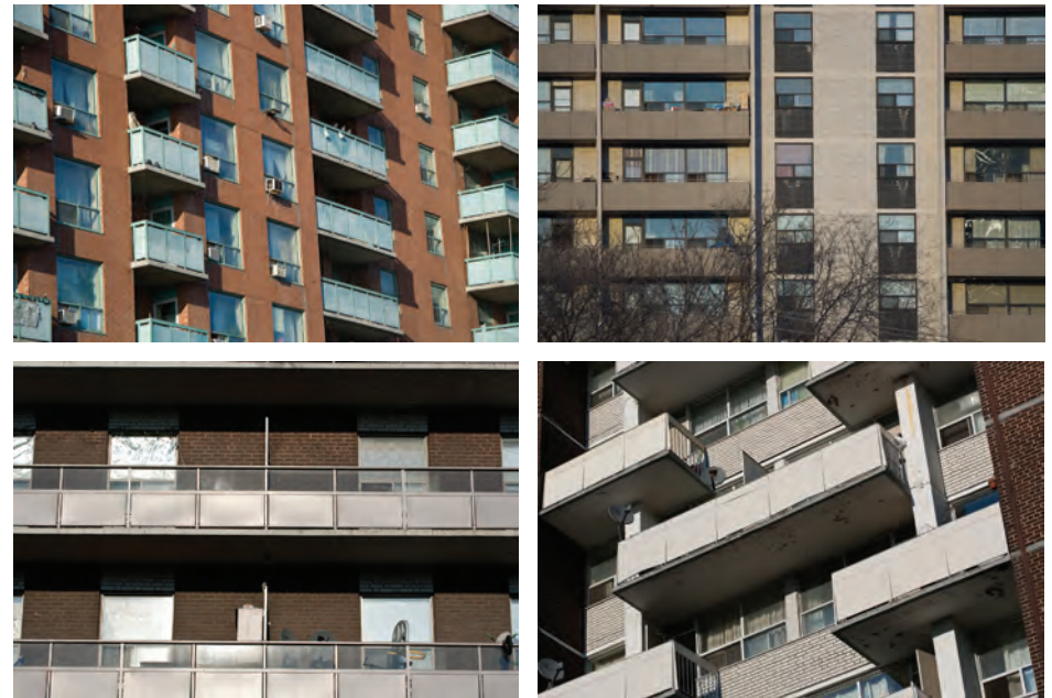
Figure 7.26. Tower balconies come in a variety of types and arrangements that will challenge the design of pleasing and performative balcony enclosures. [Photos: Jesse Colin Jackson.]
