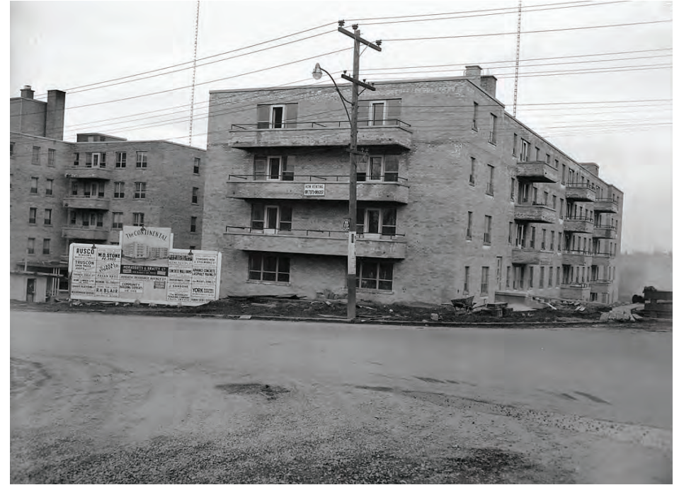
Figure 4.3. Example of an apartment building ranging from 4 to 5 storeys in response to the sloped site. These sorts of contextual idiosyncrasies make it difficult to establish clear classification systems. This building features both single and double balconies, with combined masonry and steel tubing guard. Within less than a decade, the open shared balcony gave way to balcony dividers in the form of opaque, person-height privacy screens. [Source: City of Toronto Archives.]
