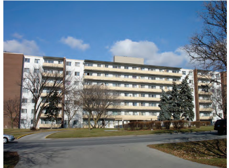
Figure 7.33. This apartment building has two types of balconies. The single balconies serve one suite and have one side enclosed by the projecting shear wall. The long, grouped balconies have metal dividers separating the balcony space allocated to each of the suites sharing the balcony.
