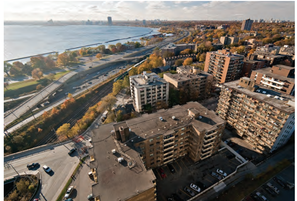
Figure 7.2. Entire neighbourhoods can be revitalized and made more sustainable through tower renewal projects that address the key attributes of comprehensive building retrofits, and bring this housing stock into the 21 st century. [Photo: Jesse Colin Jackson.]
