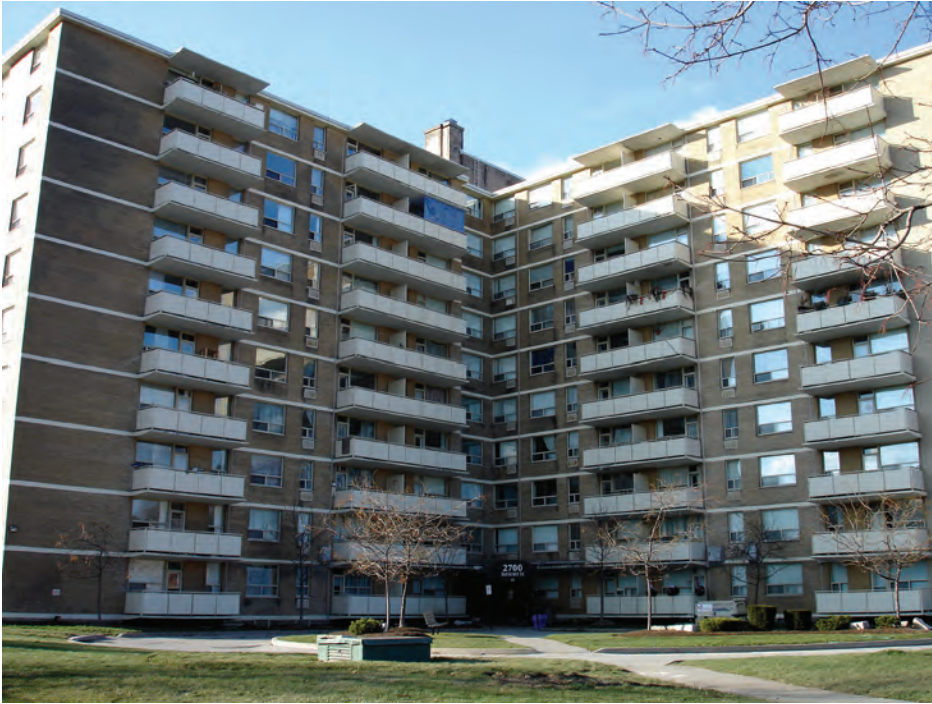
Figure 7.40. This L-shaped apartment building has a combination of single and double balconies. The double balconies are divided with metal partitions that would have to be replaced when the balconies are enclosed with tight fitting, fire-rated separators.
