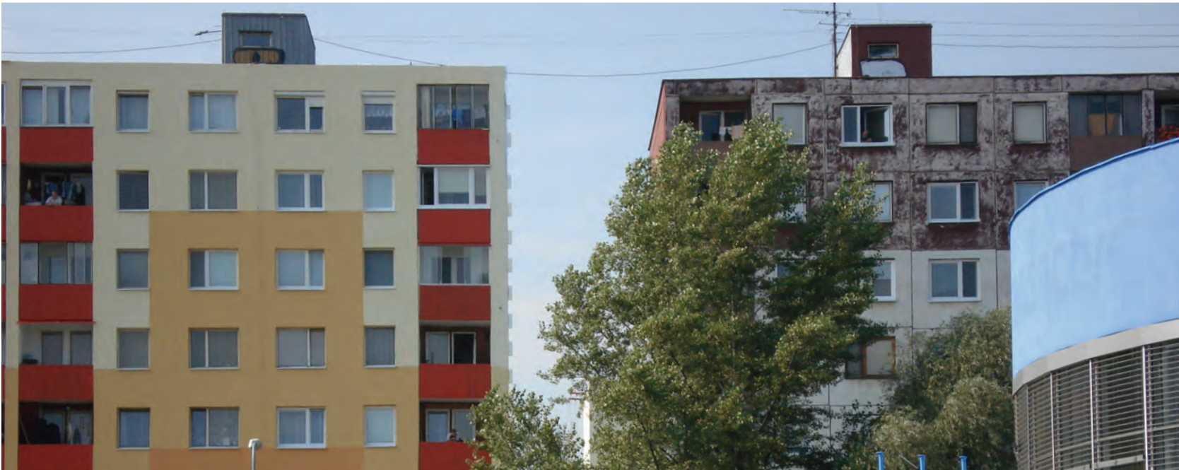
Figure 1.19. In Bratislava, the entire district of the Petržalka, consisting of hundreds of tower blocks, is in the process of being over-clad as part of Slovakia's environmental agreement in joining the EU. Paid for in part by the EU Commission of the Environment, the municipality, and private investors (who gain development rights on adjacent properties), the project is not only making buildings more efficient, but is also breathing new life into this aging district through new mixed use and improved public space.
