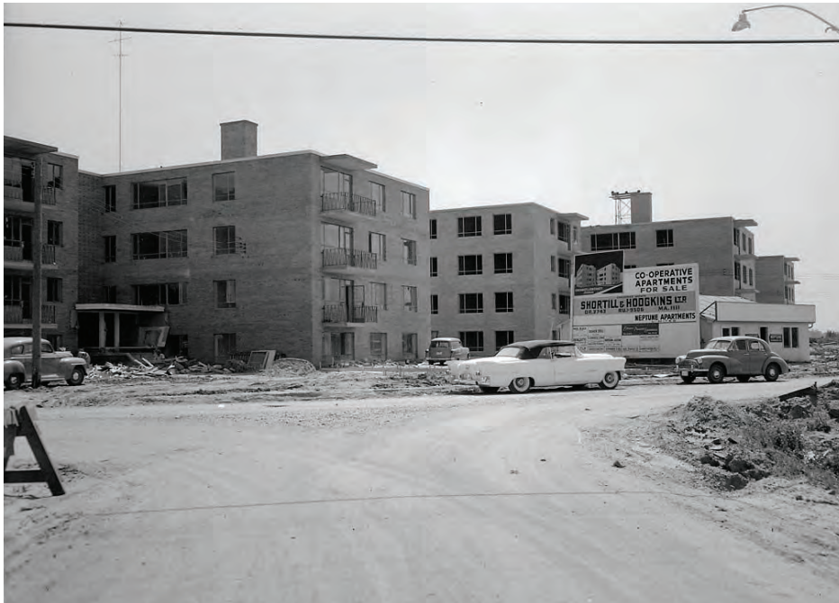
Figure 4.2. This 4-storey, 1950s apartment building has a hybrid steel and reinforced concrete structural system, and a brick veneer cladding. Operable windows are the only means of ventilation and there is no elevator service. Technically, it is not classified as a mid-rise apartment building, but unofficial estimates indicate this typology may be more prevalent than high-rise apartment buildings, based on the number of units or suites. Note the use of the cantilevered floor and roof slabs for balconies and awnings. [Source: City of Toronto Archives.]
